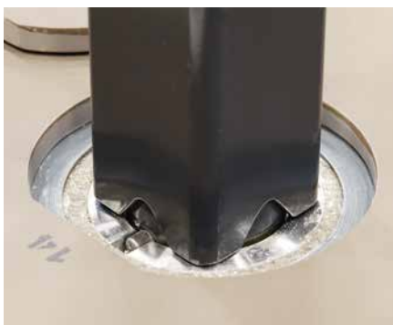
Pfosten in Bodenhülse
